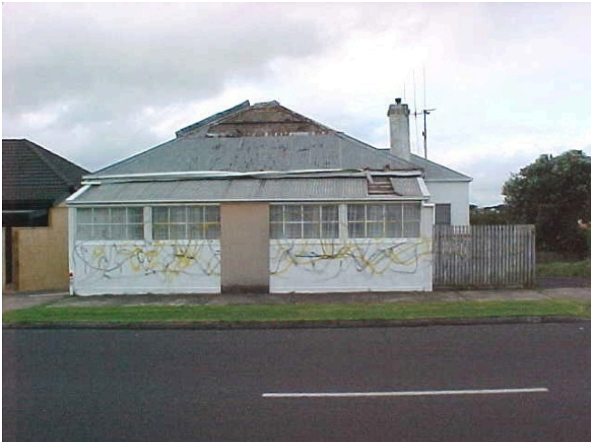
94 Merri St. 2008 – showing graffiti, front door removed and part of roof demolished. Photo courtesy of Heritage Victoria website.
