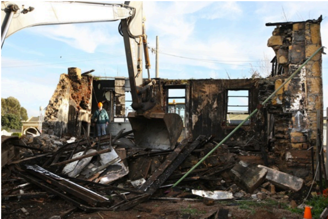
Day of demolition for 94 Merri St – August 6, 2011 – photo courtesy of Warrnambool Standard.
