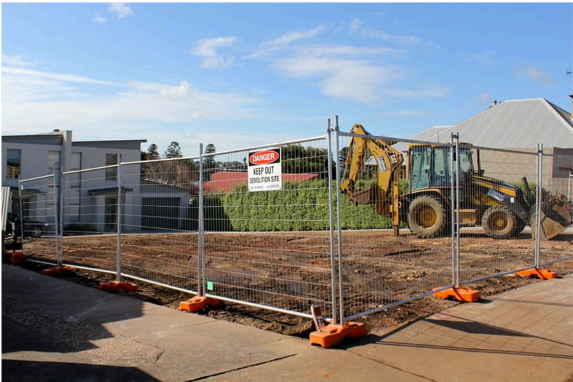
94 Merri St following demolition - August 6, 2011 – photo by Jeremy Lee ABC South West Victoria
